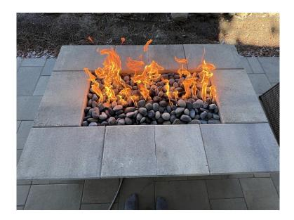
6. If desired, glue the caps in place with a heavy-duty exterior block adhesive (sold separately).
