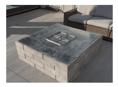
4. Place the block caps so there is approximately a 3" gap all the way around. You will have 4 caps that are cut to a shorter width. Each long side of the fire pit will have 2 of these shorter caps placed next to each other in the center. Fill inside with lava rock or fire glass.
